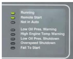
The operator panel includes a series of LED indicating lamps to allow the operator to view the general status of the generator set. Functions displayed include:
